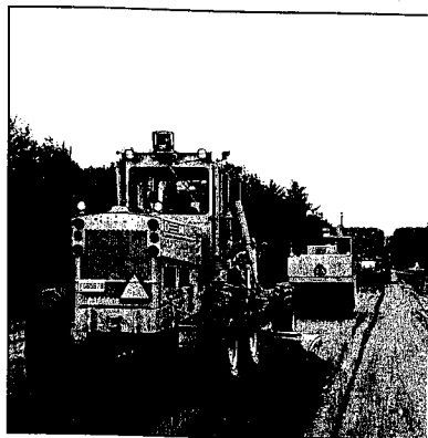
A pneumatic roller and motor grader are used to compact and reshape the pavement during a pulverization/Foamstab project
