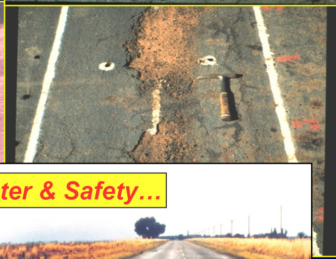
Surface Disintegration...
