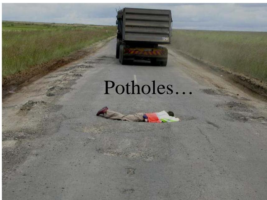
Figure 2. Failure of a secondary provincial road in Mpumalanga, not designed to carry this type of traffic.
