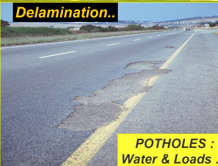
Surface Disintegration...
