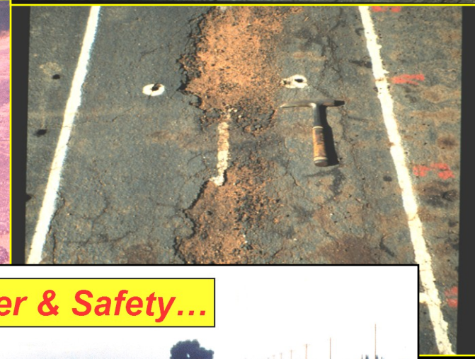
Surface Disintegration...
