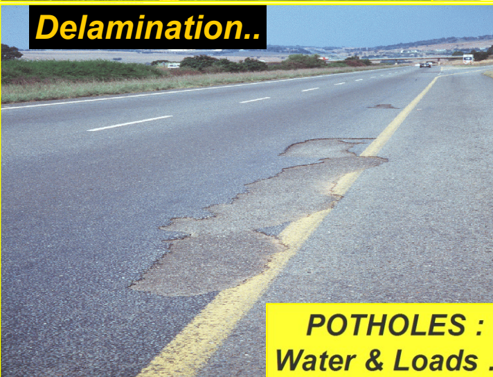
Surface Disintegration...
