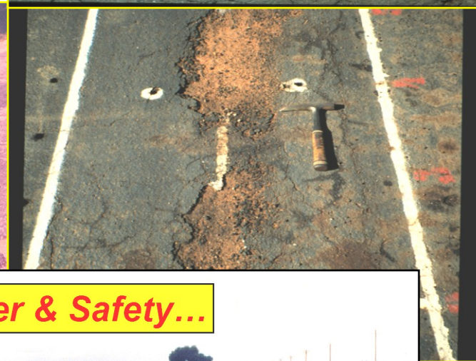
Surface Disintegration...
